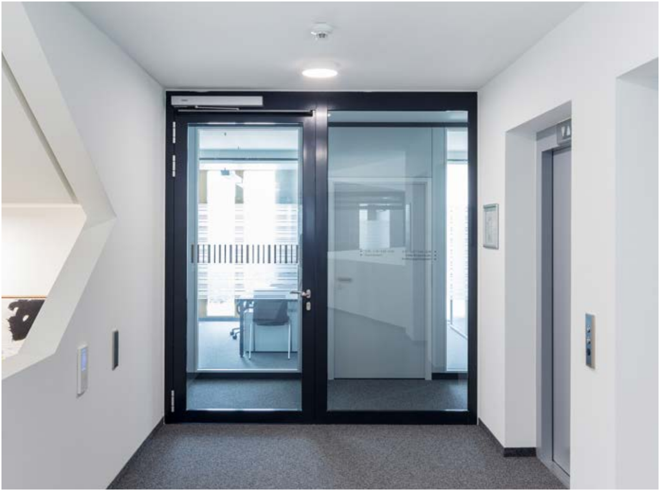
Powerturn swing door drive F/R with LS 990, Rathaus Leonberg, Germany (photo: Jürgen Pollak / GEZE GmbH)
