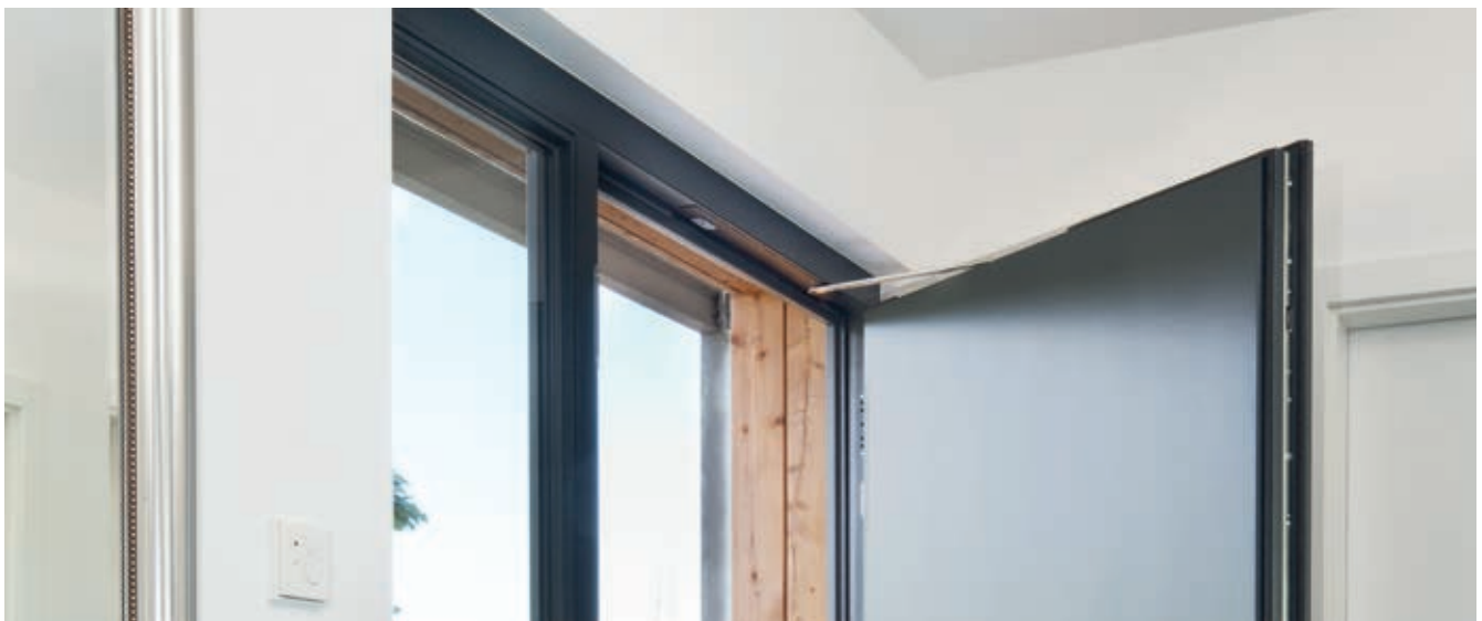
Front door, private residence, Stuttgart, Germany (photo: GEZE GmbH)
