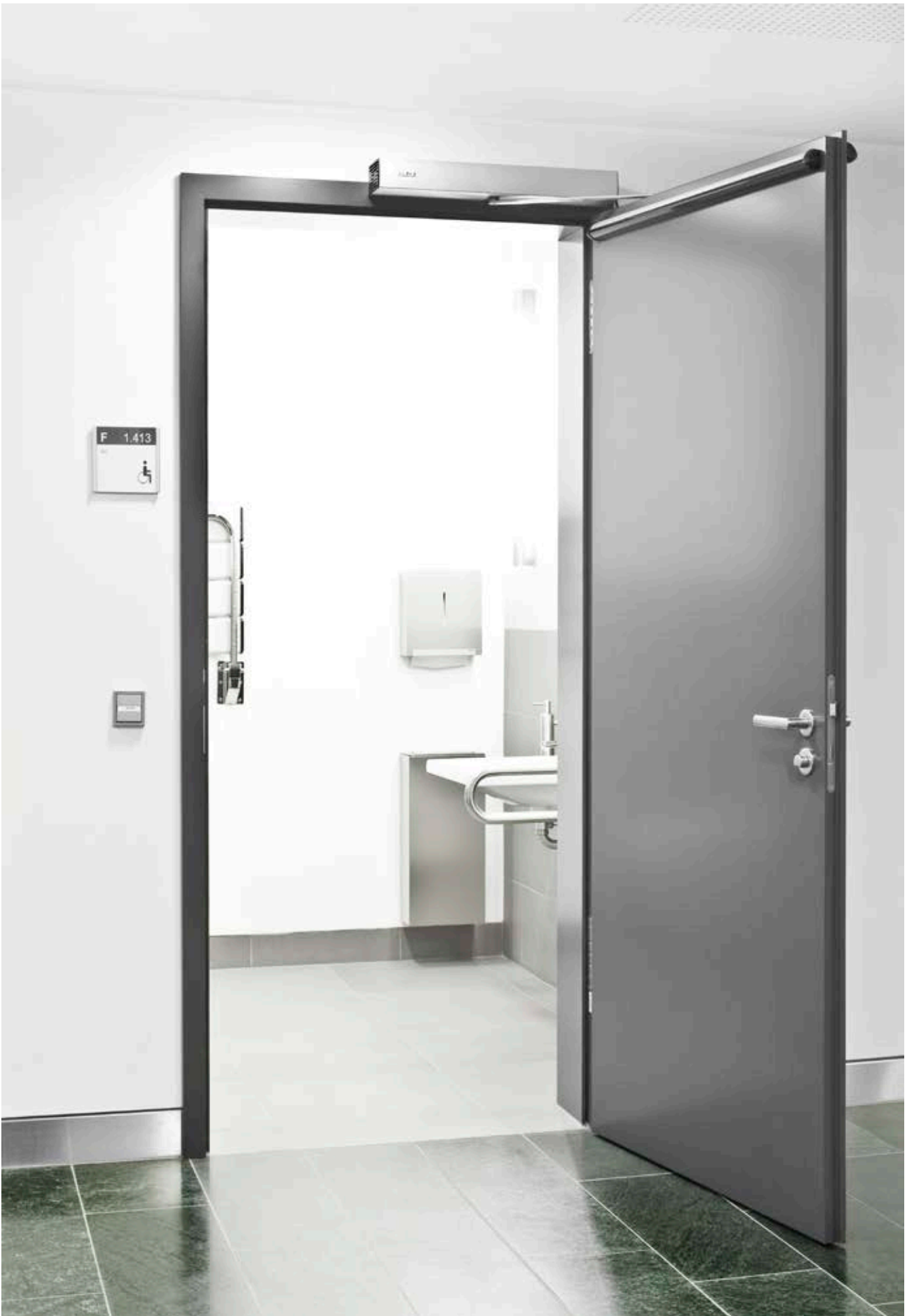
Slimdrive EMD-F swing door drive with GC 338 sensor strip, VGH Versicherungen Hanover (photo: Lothar Wels / GEZE GmbH)
